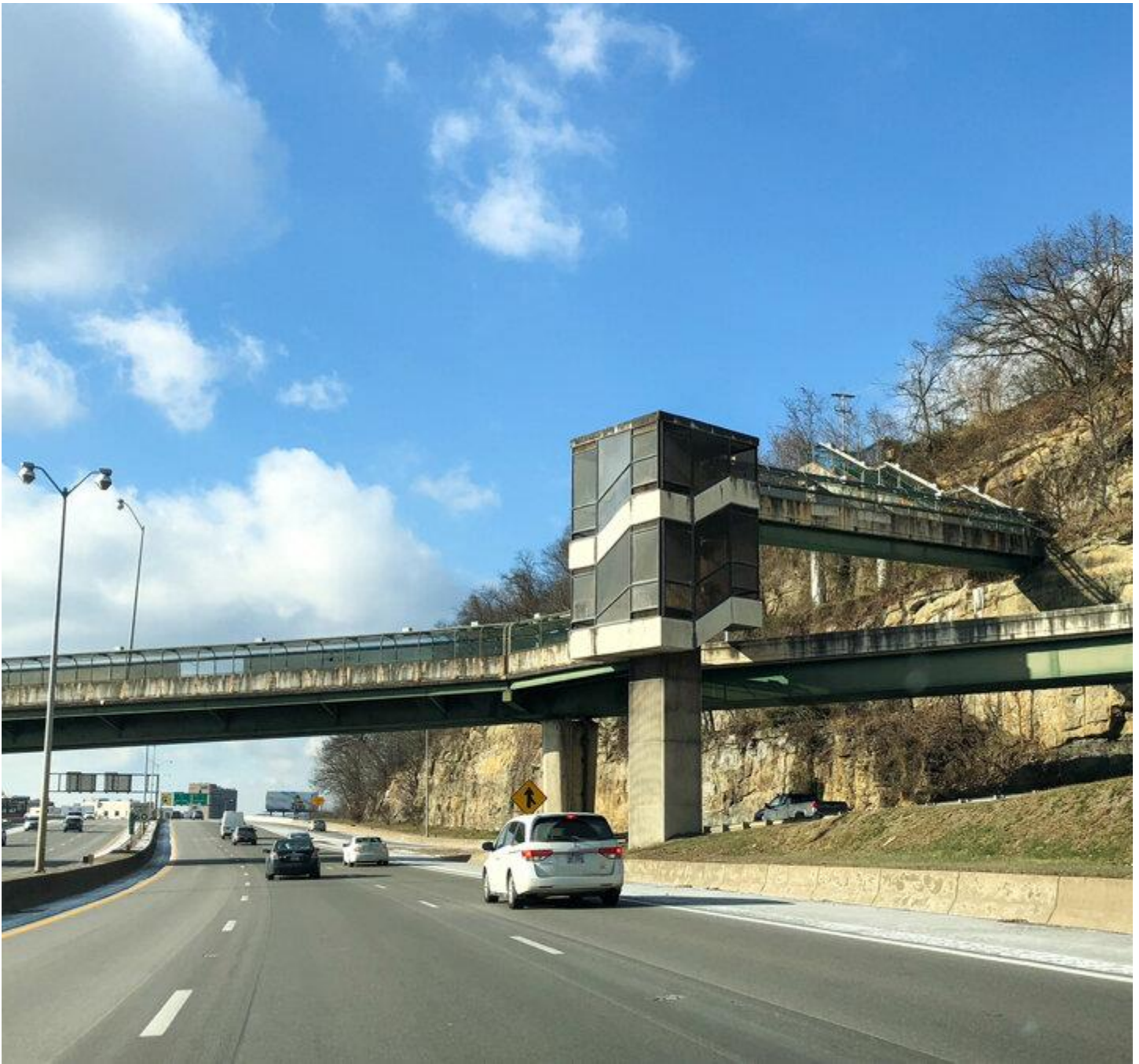
- Charleston's overpass walkways as seen from the interstate.
