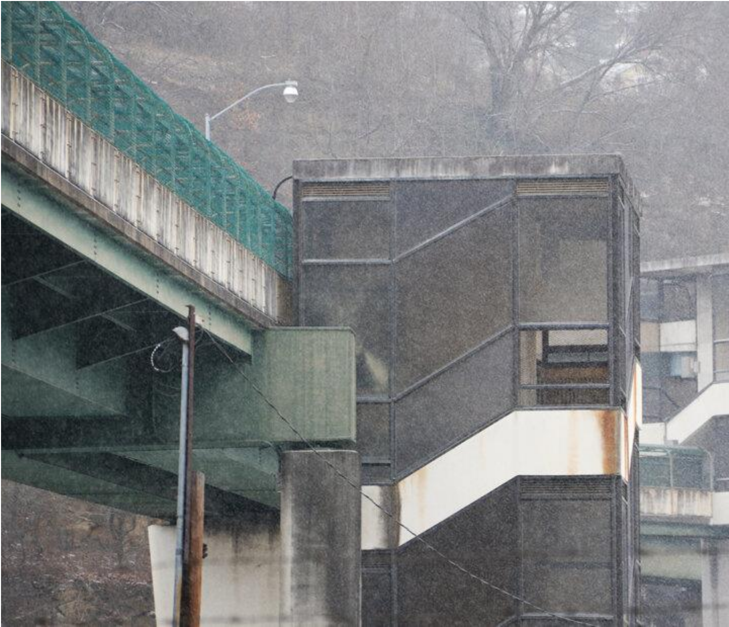
- Towers 2 and 3 as seen from tower 1.
