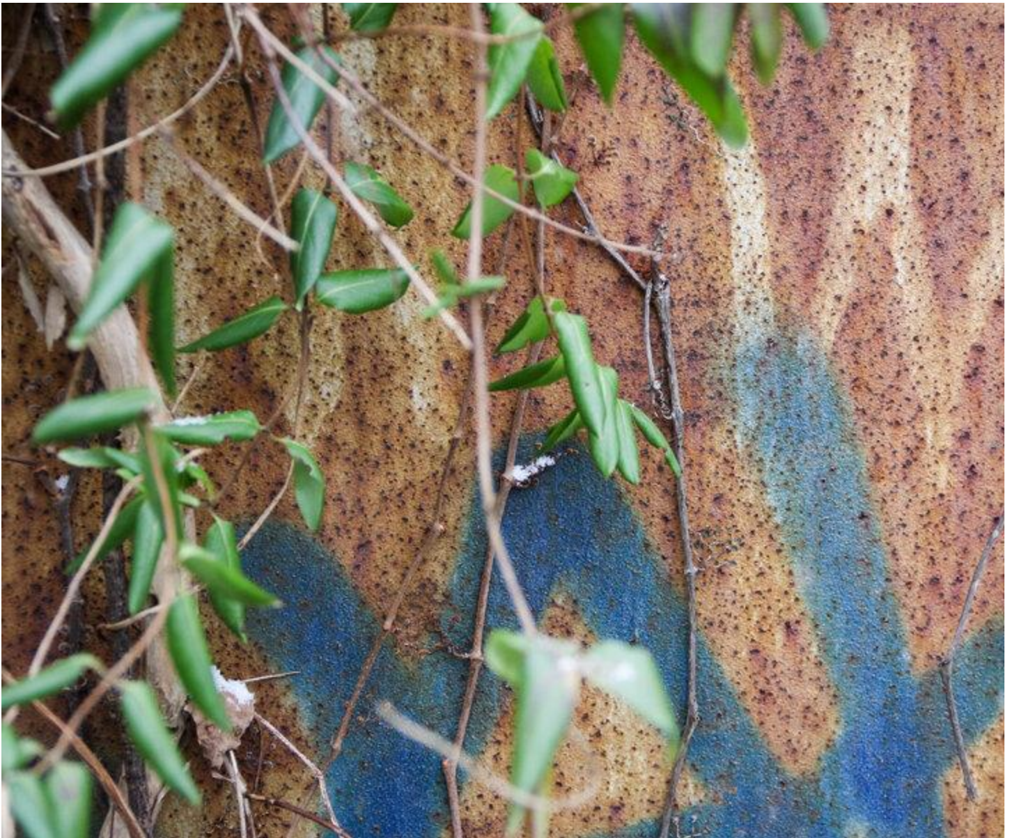
- Detail of the metal keeping the walkway from being used.
