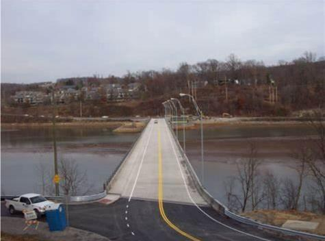
The Ices Ferry Bridge project involved the replacement of a steel through-truss bridge with a new 960-LF four-span steel girder bridge located near Morgantown, WV. The scope of work also included the construction of two retaining walls and new approaches on each side of the bridge. The new bridge spans the Cheat Lake Reservoir, a popular resort area in West Virginia.
