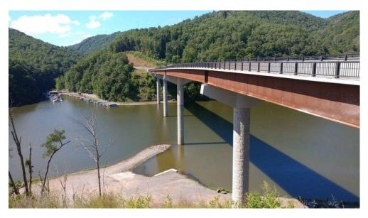
The Lilly Bridge project involved replacement of a cantilever truss bridge with a new 1,220-LF five-span, fabricated steel girder bridge. Carrying WV RT 20 traffic over the Bluestone Lake, the new bridge was erected adjacent to the existing structure. Brayman offered a significant Value Engineering (VE) proposal including substructure and superstructure modifications.
