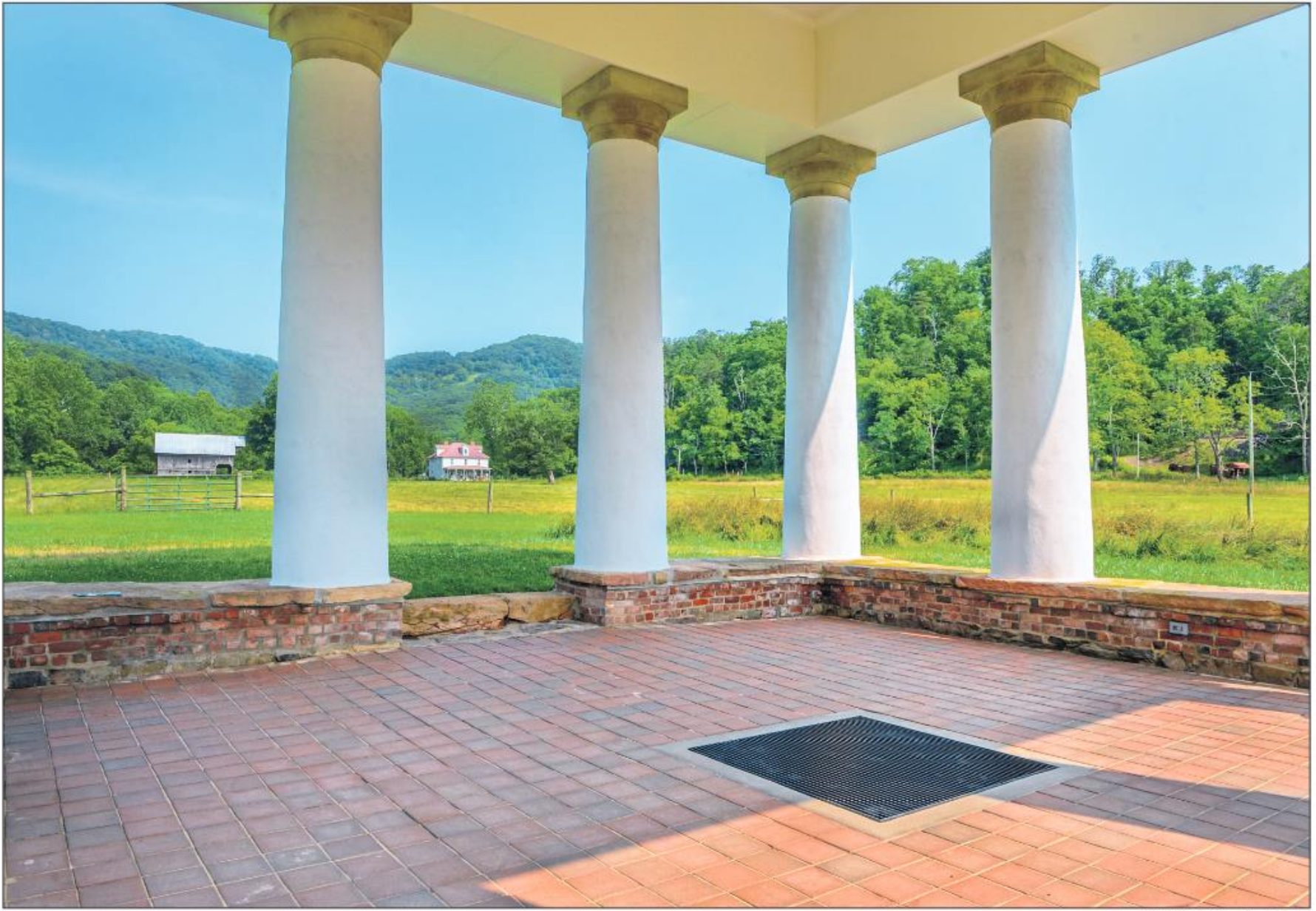
A 33-foot-square brick floor surrounds a steel grate cover the spring that once drew thousands of visitors to the Blue Sulphur Springs resort during its heyday in the mid-1800s.
