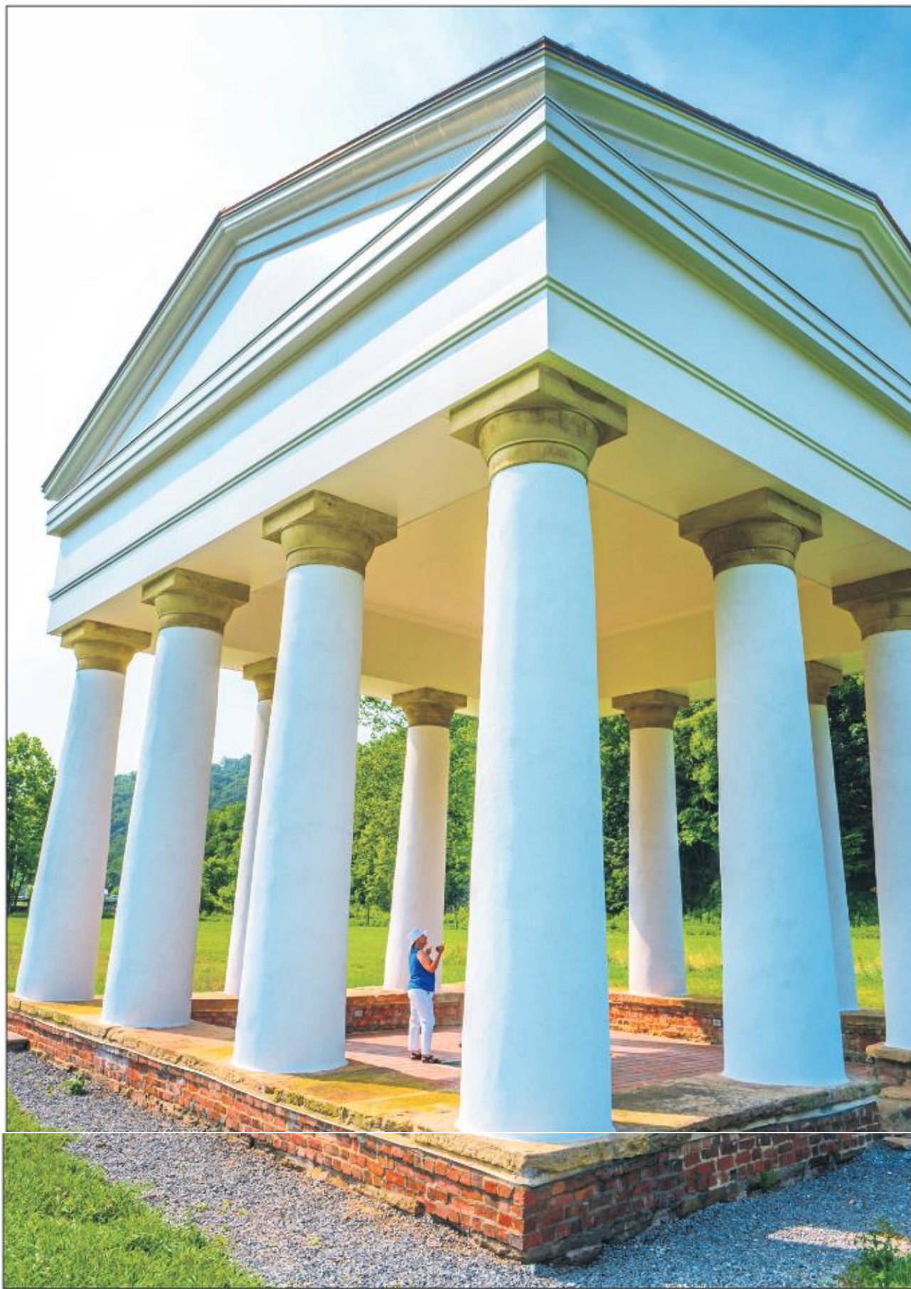
Margaret Hambrick, of the Greenbrier Historical Society, is dwarfed by the restored pavilion’s columns and roof.
