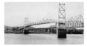
The Silver Bridge was an eyebar-chain suspension bridge built in 1928 which carried U.S. Route 35 over the Ohio River, connecting Point Pleasant, West Virginia, and Gallipolis, Ohio. Officially named the Point Pleasant Bridge, it was popularly known as the Silver Bridge for the color of its aluminum paint.
