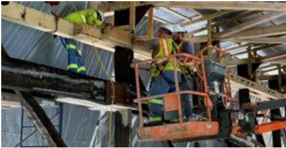
Work on the bridge has been taking place for months. (Photo/WVDOH)
