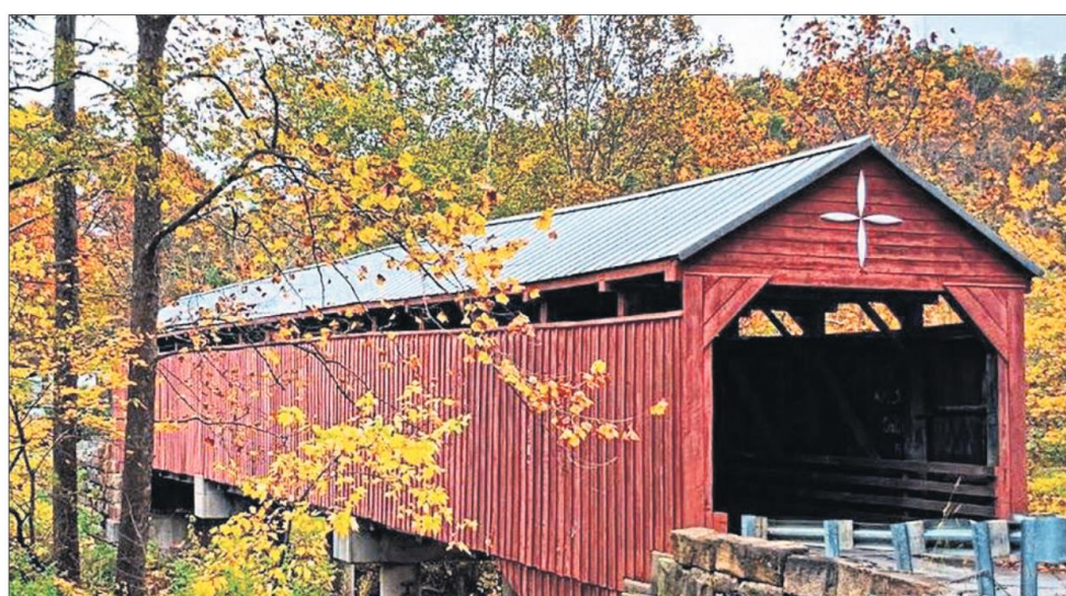
The Carrollton Covered Bridge is seen before being damaged by fire in 2017.
