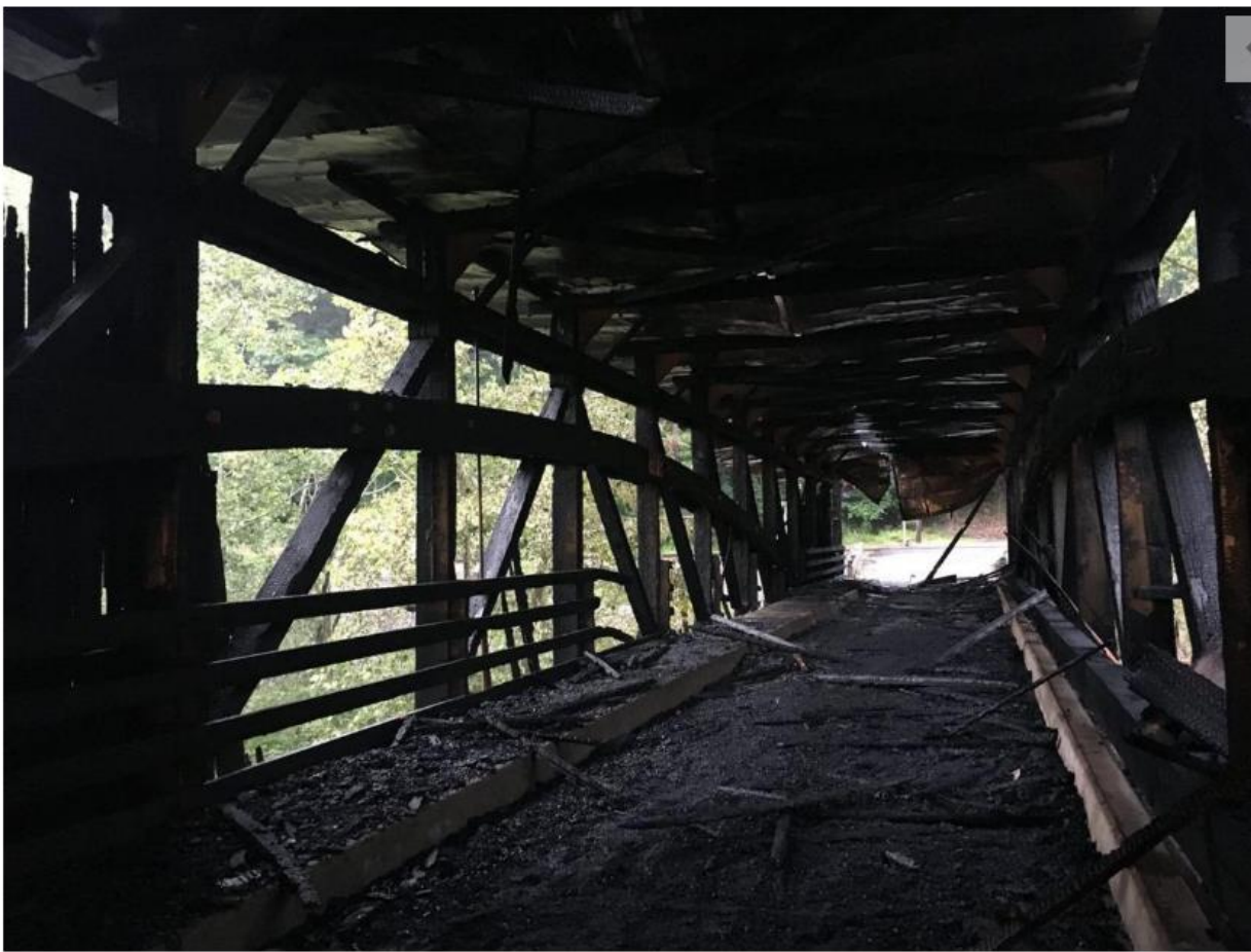
A view from the interior of the bridge shows charred wood atop its concrete deck, added in 1963.
