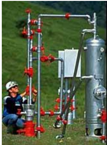
Natural gas from underground formations flows through pipes on the surface sometimes called a "Christmas Tree." Photo: NGSA
