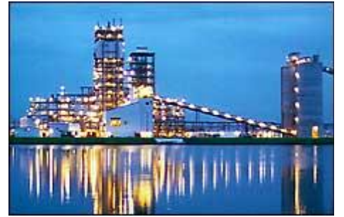
One of the most advanced - and cleanest - coal power plants in the world is Tampa Electric's Polk Power Station in Florida. Rather than burning coal, it turns coal into a gas that can be cleaned of almost all pollutants.
