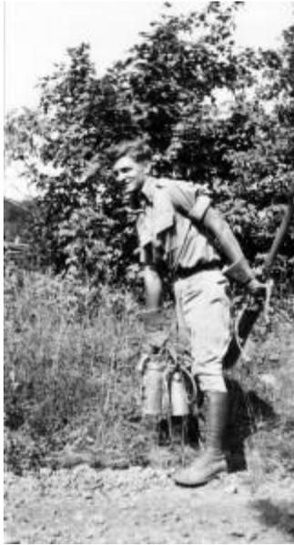
*Leonard Swing prepares to use a shovel to bury seismic recording devices known as pickups or jugs. Formally known as seismometers, the jugs were used with a time-recording instrument (a seismograph) to map the subsurface in the 1915-1940 era. Photo courtesy of WVONGA*
