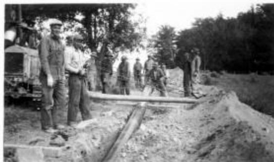
*A pipe-laying crew pauses for the camera in the 1915-1940 era. They got the job done with a bulldozer (far left), chains, cables and elbow grease. Photo courtesy of WVONGA*
