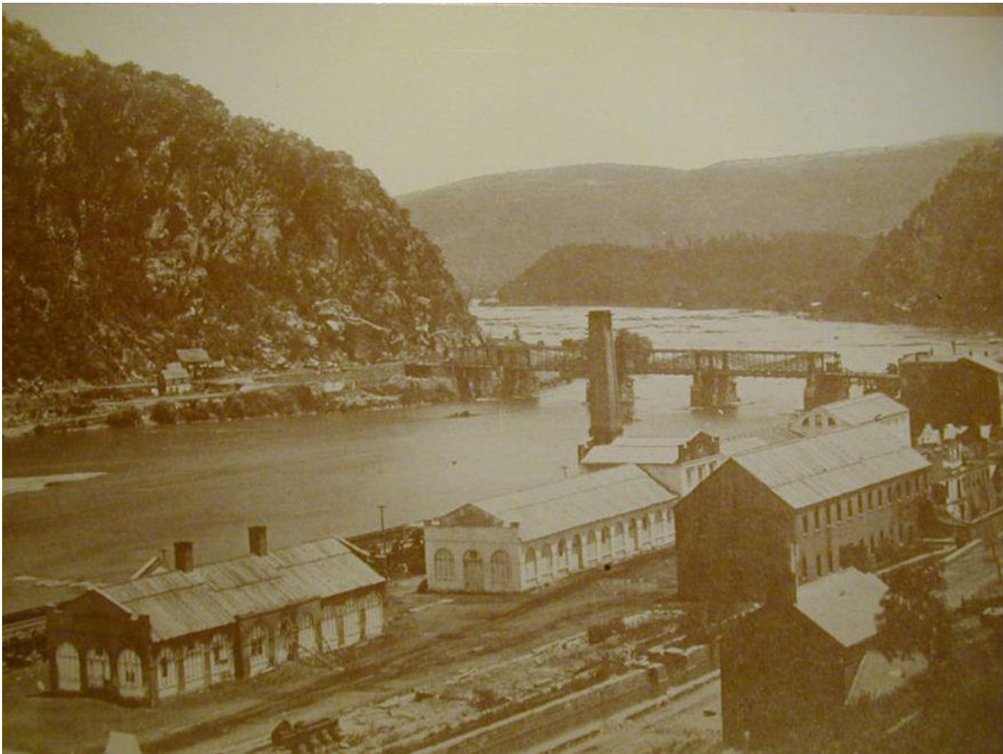
Ruins of the U.S. Armory on the banks of the Potomac River at its junction with the Shenandoah River, Harpers Ferry, Virginia during the Civil War. The B&O Railroad bridge across the Potomac River is at top center, destroyed and rebuilt 9 times during the Civil War.
