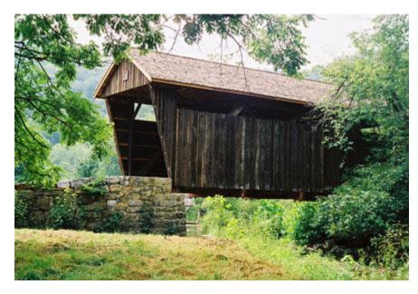
One of the most photographed in the state, this Monroe County span is located not far from the Laurel Creek Bridge, north of US 219. Owned by the county historical society and open to pedestrians, it was part of the White and Salt Sulphur Springs Turnpike. A Long truss built in 1903 by Ray and Oscar Weikel (ages 16 and 18 years old) and E.P. and A.P. Smith, it is more than 11.5 feet
