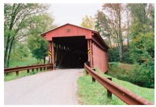
Built by R.B. Cunningham and G.W. Staats in 1890, this Long truss bridge carrying Jackson County 21/15 over Left Fork of Sandy Creek near Sandyville was dismantled and relocated 1924. The 11.75-foot-wide, 101.25-foot-long span also received some repairs in 1979.
