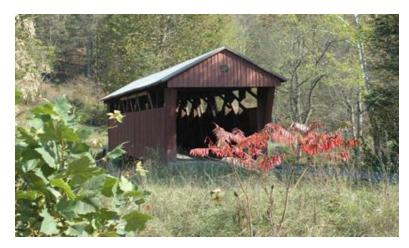
This 12-foot-wide, 81.5-foot-long Long truss, built in 1899 carries Greenbrier County 62 over Second Creek. While originally costing only \$200, renovations in 2001 by Allegheny Restoration & Bldrs, Inc. of Morgantown, WV totaled \$391,646.
