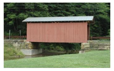
Located on Wetzel County 13 near Hundred, this kingpost truss is 12.75 feet wide and 36 feet long and still carrying traffic. Few details of its 1880 or 1881 construction are known. Lone Pine Construction, Inc. of Bentleyville, PA completed renovation of the bridge in 2001 for \$218,409.
