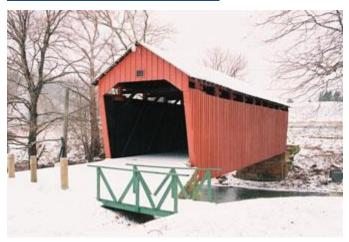
A 14.25-foot-wide, 75-foot-long multiple-kingpost truss, this covered bridge built for \$1483 by Asa Hugill in 1881 once carried the traffic of Harrison County 24/2 near the northern edge of Bridgeport.
