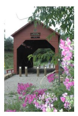
Nearly 13 feet wide and 40 feet long, this bridge was completed in 1889. W.A. Loar built the abutments and William and Joseph Mercer built the superstructure, using a kingpost truss. The bridge is located on Monongalia County 43/3 north of US 19 near Westover. A contract for repairs to the trusses, new floor beams and deck installed was awarded to Hoke Brothers Contracting, Inc. of Union, WV for \$185,684.
