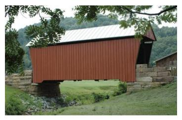
This 12.5-foot-wide, 42-foot-long Long truss built in 1889 by John Ash and S.H. Smith crosses Pike Fork of McElroy Creek just east of WV 23 in Doddridge County. No longer carrying traffic, the bridge underwent \$353,697 worth of renovations by The Righter Co., Inc. of Columbus, OH in 2002.
