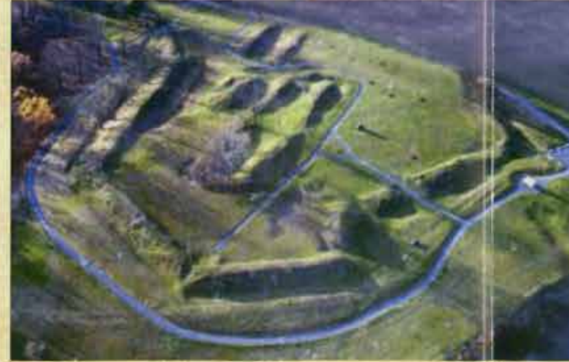
Fort Mulligan - Federal or Confederate troops occupied this hill and its surrounding area beginning as early as August 1861.
